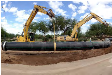
Infrastructure placement and upgrades
