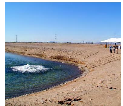
SRP's Superstition Mountain Recharge Project (underground water storage)
