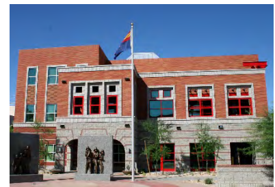
Chandler's Fire, Health, and Medical Department headquarters
